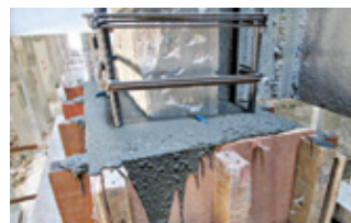
Micro Concreting
