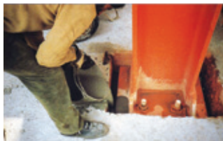
Non Shrink Cement Grouting
