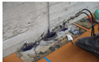
Epoxy Grouting
