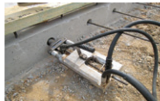
Cable Grouting
